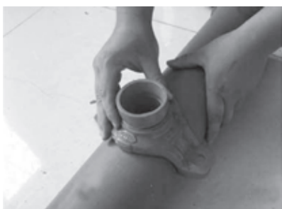
4. Install the Mechanical Tee in the hole.
