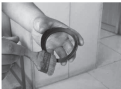
2. Spread lubricant on gasket ring.
