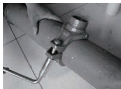
6. Secure the nuts and bolts of side outlet from both side.
