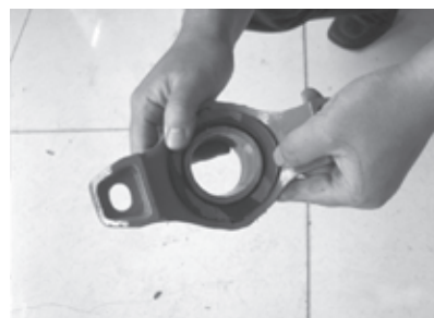
3. Put gasket seal in the Mechanical Tee.
